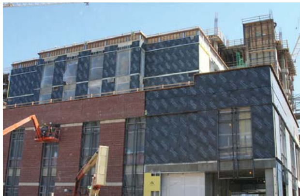
Windows and bricks have been installed on the west side of the new Le Bonheur hospital. When it opens in summer 2010, it will feature 12 floors.
